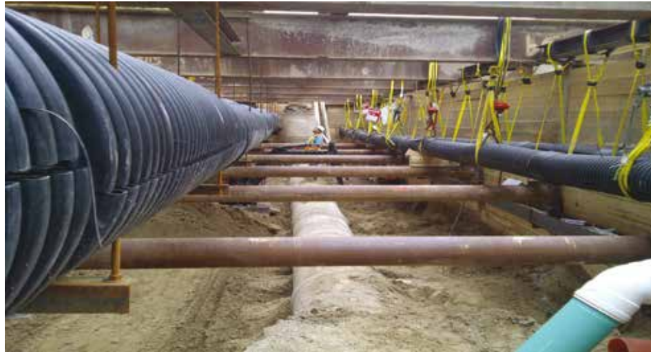
Utility coordination efforts on the TTC Union Station Expansion Project.
